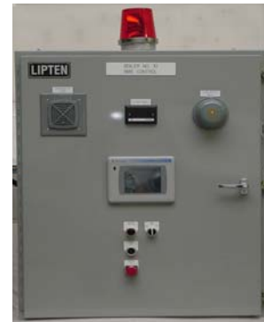
New COMBUSTION PAC control panel
