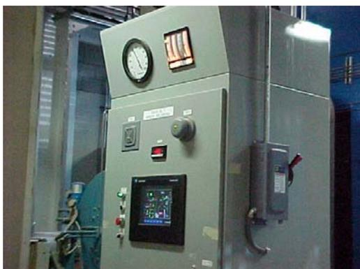
A independent ultraviolet and/or infrared flame switch is employed to add further redundancy to the safety circuits. A color touchscreen display (HMI) is mounted on the door of the enclosure giving access to all boiler operating controls and allows monitoring of all critical parameters.
