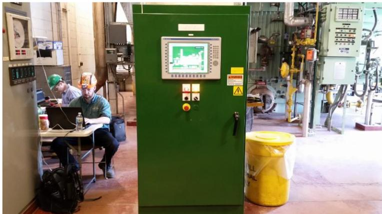
Replacing an old analog boiler control system with advanced PLC controls is usually not a challenge, except when it has to be done in only one week. That was the challenge Lipten faced this summer when providing a control system upgrade to Boiler #2 at Neenah Paper's Stevens Point, WI facility known as the Whiting Mill.
