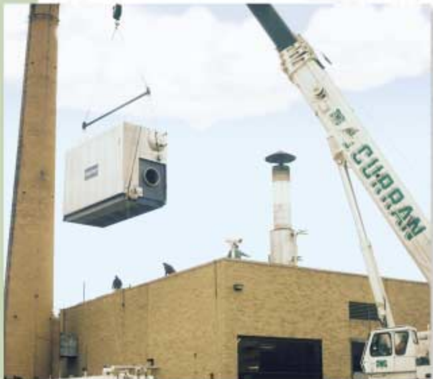
High efficiency replacement boiler for a medical center.
